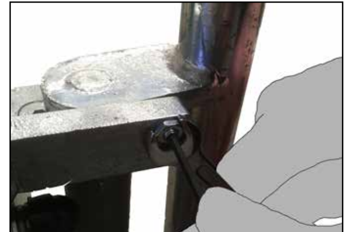
N. Using a M6 spanner and 4mm hex key, slacken off the locking nut and adjust the grub screws so that the gate leaves meet in the middle. Once centre position is correct, lock off grub screw using nut.
